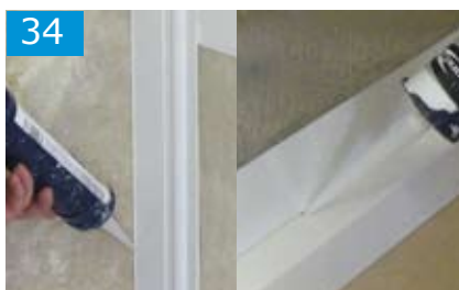
IMPORTANT: Seal all joints between compensators, walls, panels and shower tray or floor, on the inside and outside of the shower area using silicone sealant.
