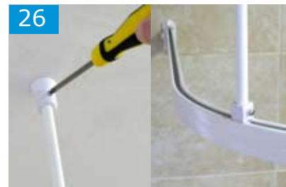
Secure drop rod into ceiling rose and rail connector into the top side of the curtain rail by tightening their respective fastening screws.
