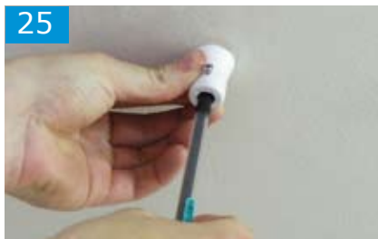
Mark position for ceiling rose and fix to ceiling using a suitable fixing (not supplied). Cut drop rod to length.
