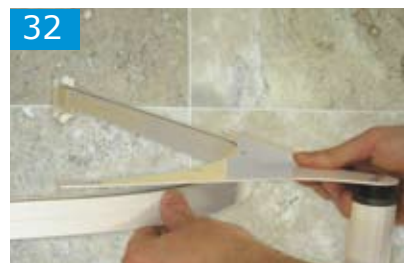
Place boomerang bracket in the top of the post, pilot drill holes in the rails top channel and fix to the post through the pre-drilled holes. REMOVE PLASTIC DUST COVER FIRST.
