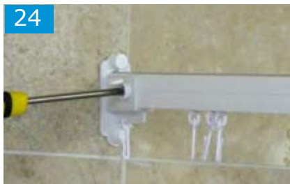
Secure curtain rail into wall brackets with No8 x 13mm pan head self tapping screws and caps.
