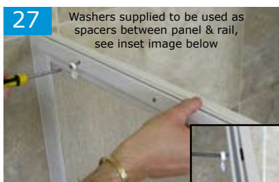
FULL HEIGHT FIXED PANEL: Fix curtain rail to panel by placing rail against the top inside edge of the panel. Drill a 3.5mm hole in panel top rail & post through curtain rail. Fix rail to panel with No8 x 25mm screws and caps and to post using No8 x 38mm screw, as in Step 30.
