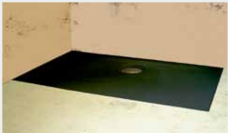
Make existing floor and Eco-dec® absolutely level
