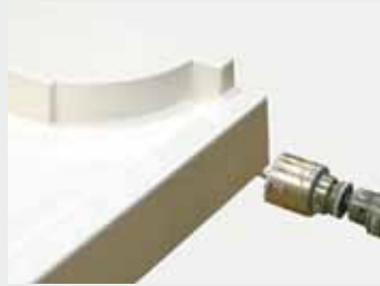
Position the waste pipe to suit
