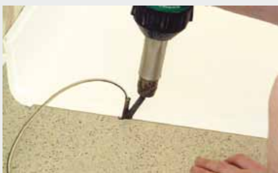
Hot seam weld flooring to the Swift
