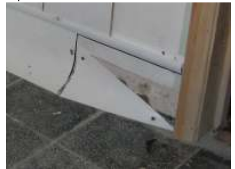
Secure the bottom edge of your cut-out to floor. You should now have a tapered profile finishing at the door
