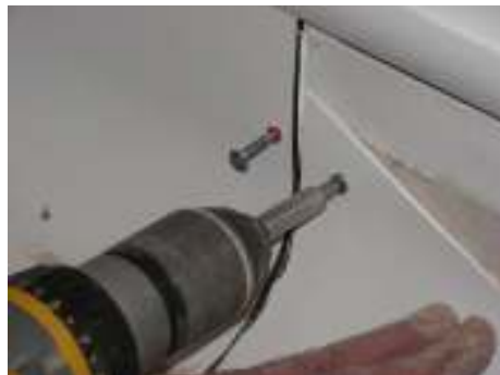
Screw the coving and the top edge of the cut-out to the wall.
