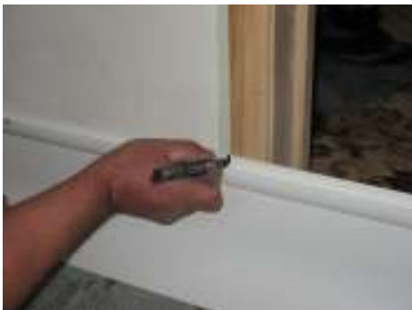
Contour coving can be easily modified to finish at a door architrave. Mark the size required
