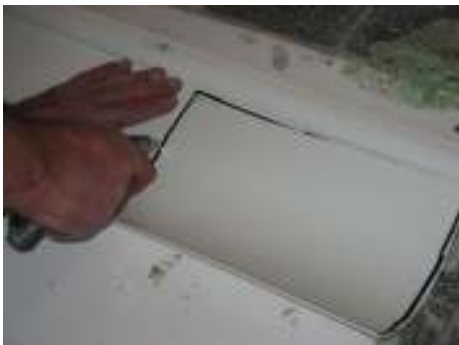
Measure back approximately 300mm from the architrave towards the corner and mark and cut out a rectangle.
