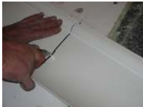
Cut to length using a Stanley knife
