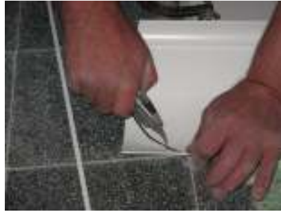
Carefully cut away the outer extremity of the coving so that it will butt up tight in the corner
