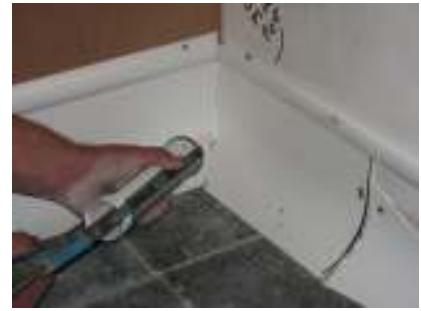
Use silicone sealant at the corner joint to form a seal between the coving sections
