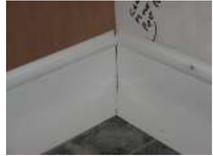
Both coving profiles should come together with a neatly cut edge
