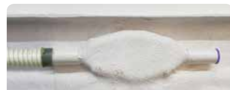
Connect the flexible pipe to the 22mm outlet & P12 waste pump. Blank off side not required.
